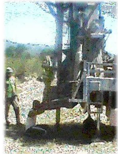
2020 – So happy - Well drilling in Natitingou
