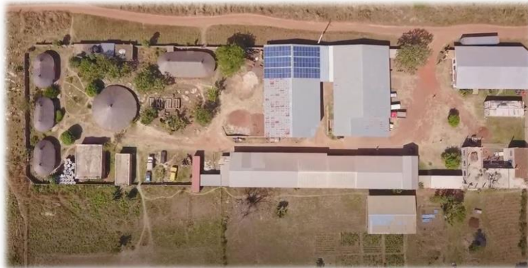
2020 – our partners for the future CFL Liweitari Switzerland
